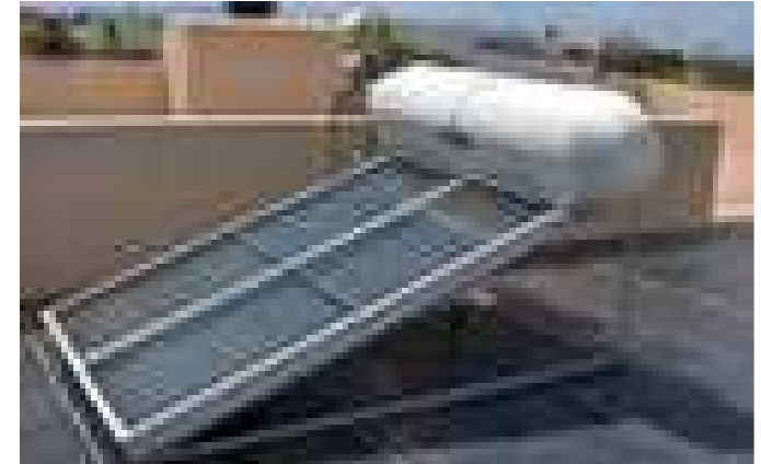
Solar Geyser on roof
